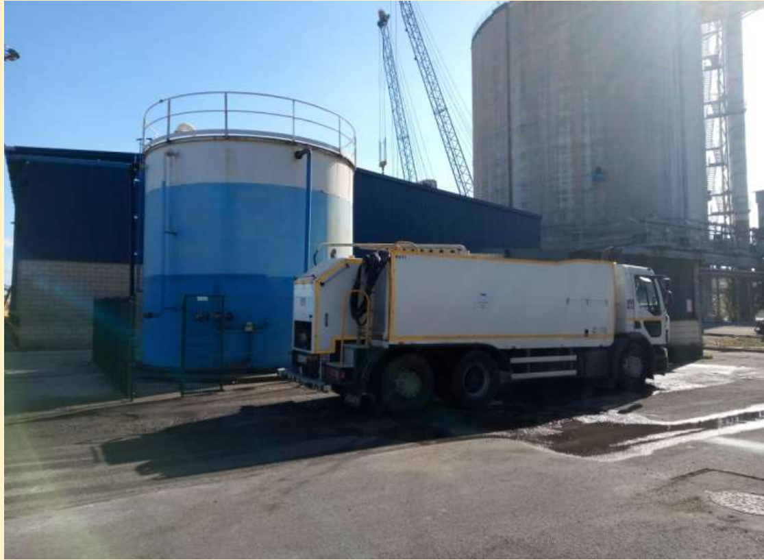
Illustrations: Rainwater deposit of 160 m 3
